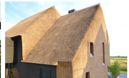
Riet in dak
